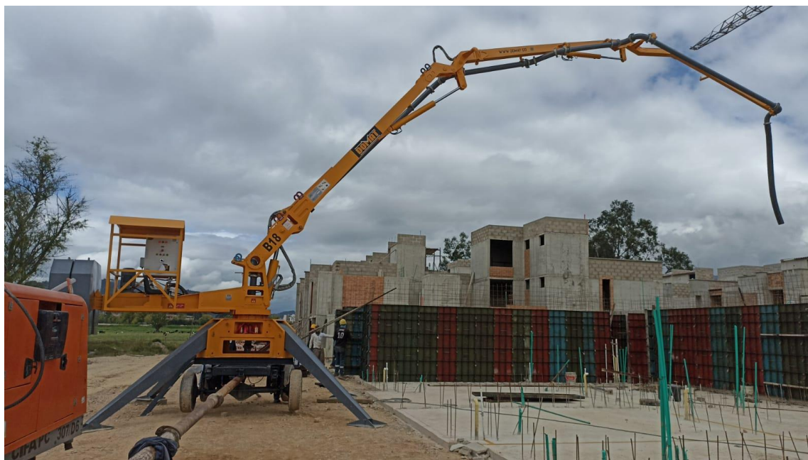
DOMAT B SERIES Hydraulic boom concrete distributor
